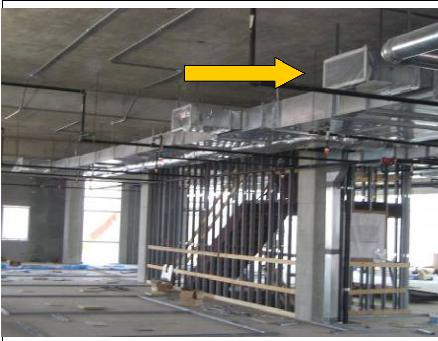
Pictured: Installed duct work is protected from construction dust.
