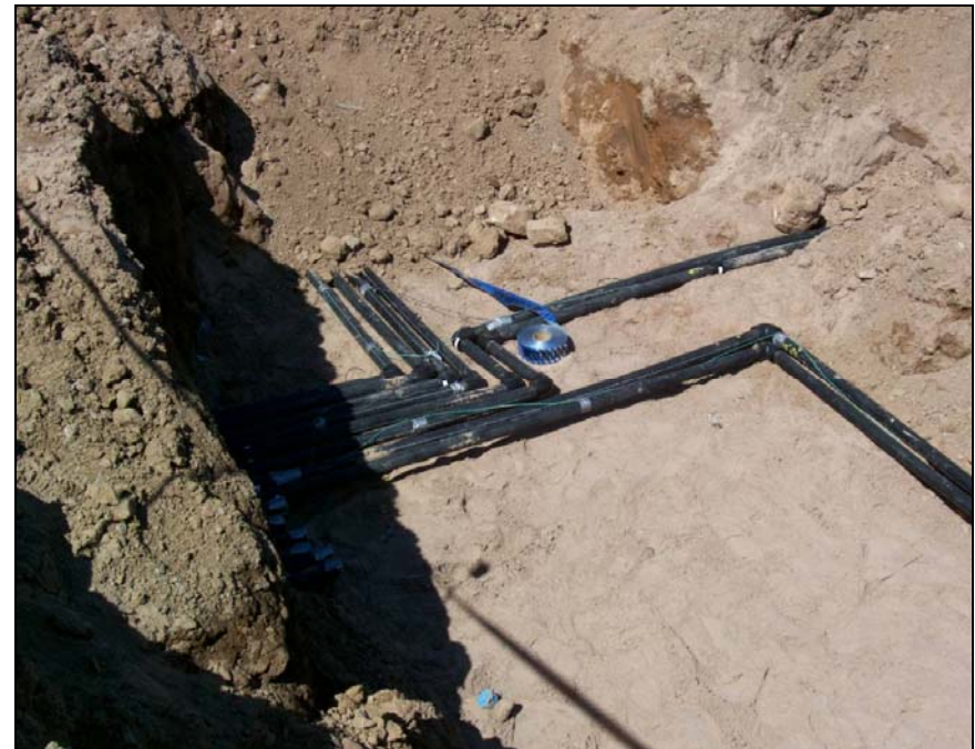
Pictured: The geothermal well during installation.
